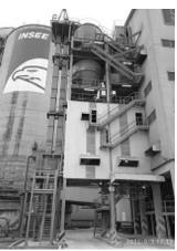
One of this project's objective is to reduce clinker factor by using Granulated Blast Furnace Slag (GBFS) and Fly Ash, with investment of 994 mio LKR. The construction phase is now completed and now in operation.  $CO_2$  reduction target is 70 kg  $CO_2$ /ton cementitious reduction.
